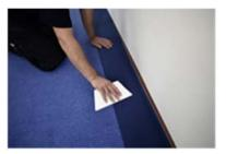
Remove fresh adhesive residue immediately with a clean white damp cloth.
