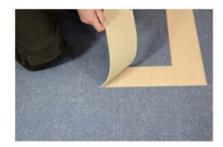
Apply a fresh layer of acrylic adhesive. Lay the Artline border into the adhesive after the appropriate waiting time specified by the adhesive manufacturer and using a rubbing board press the border firmly into the adhesive (see below).
