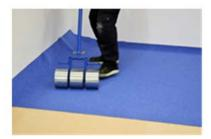
Roll the sheet or press into the adhesive with a rubbing board or glider within the open time of the adhesive.
